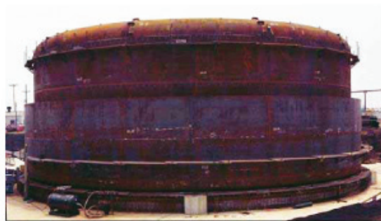
Figure 12. Type IIIA Primary and Secondary Carbon Steel Liners - Late Tank Construction
