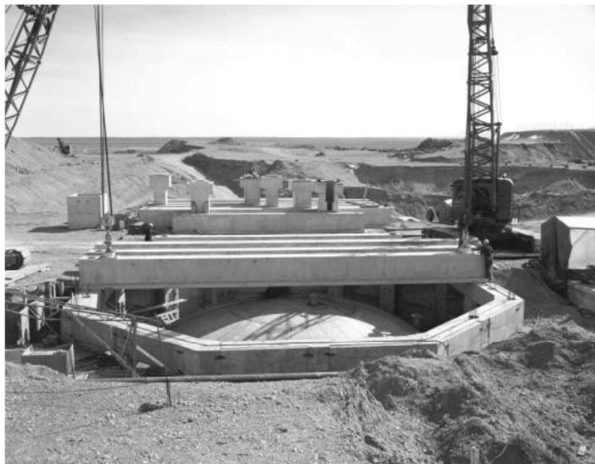
Figure 8. INL Tank WM-185 Vault Dome, Support Beams, and Risers (USDOE-ID 2003)
