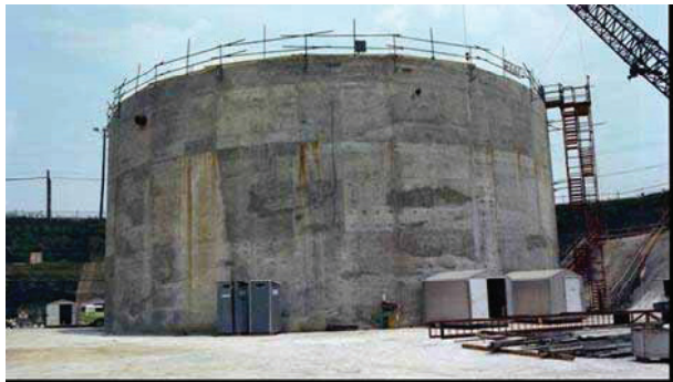
Figure 13. Concrete Vault Around Steel Tank - Final Construction of Type III/IIIA Tank
